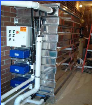
Above ground Installation
